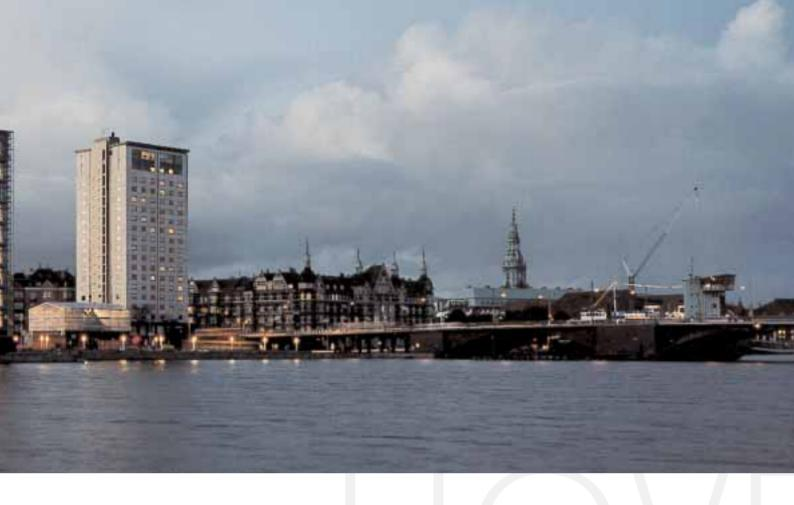
**HOVERING** The 40 metre high building seemingly hovers over the quay on Kalvebod Brygge. The Glass Cube rests on granite-clad columns which support the 57x57 metre square building. There is free passage along the harbour fairway, and the Glass Cube forms a natural end to the esplanade leading to Langebro.
